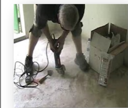
Mark Barrows applying the adhesive.
