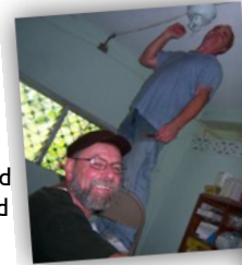
Fans being installed
